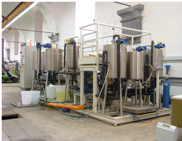
Figure 1. Comprehensive view of the experimental pilot plant.
