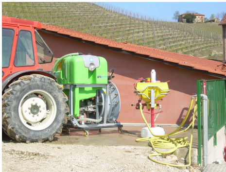
Figure 7. Dedicated paved area for loading and cleaning of sprayers, equipped with a collecting system for PPP contaminated liquids and with an independent induction hopper for loading sprayers.
