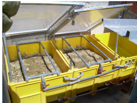
Figure 12. Biofilter installed in Fontanafredda demo farm
